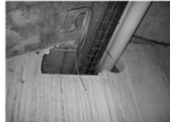
Fig. 2: Internal leakage – cable penetration to an adjacent building section (Source: IngBEU)
