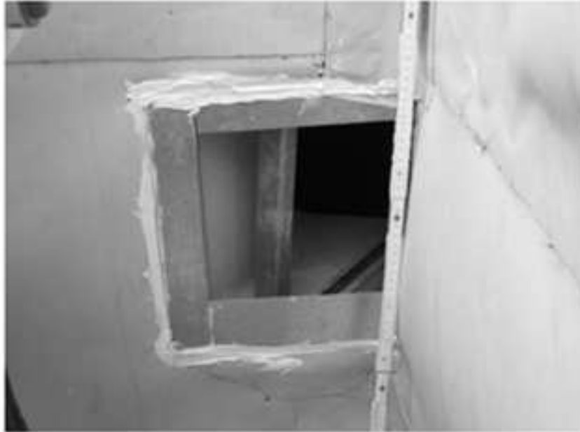
Fig. 3: Smoke outlet in an elevator shaft (Source: IngBEU)
